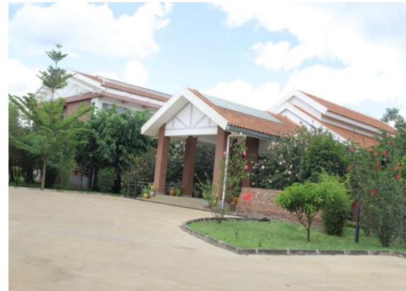
Main entrance to the research centre facility
