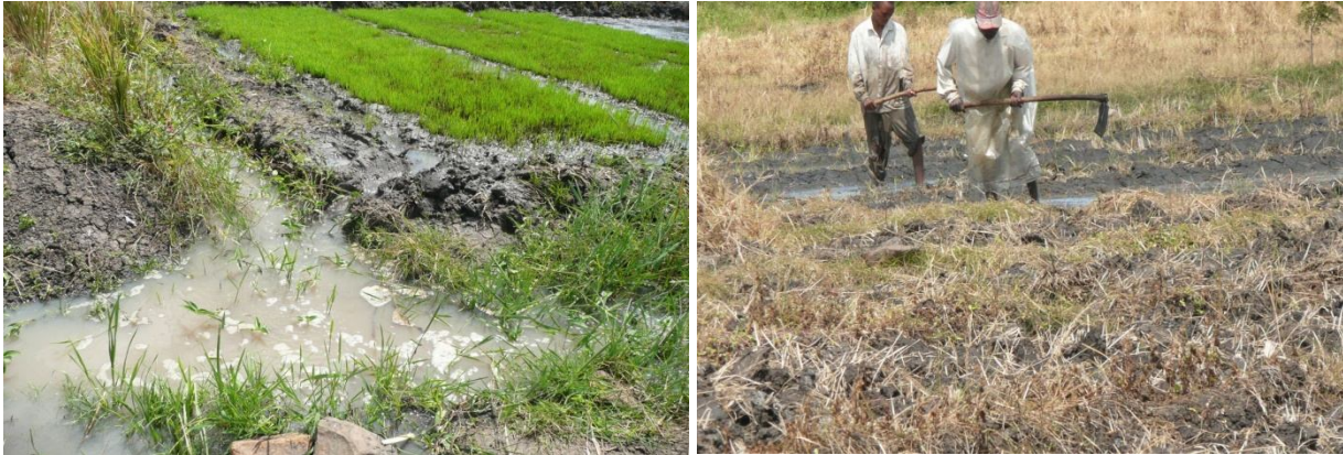
Figure 6 Excessive seepage from canals causes waterlogging in fields (photos by B. Mati)
