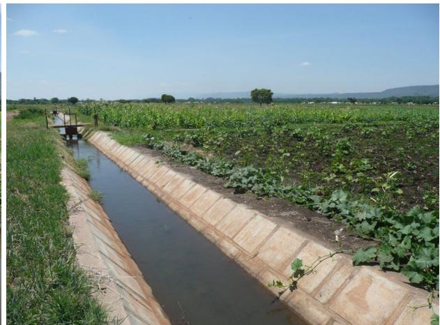
Lined canal stops waterlogging by preventing seepage
